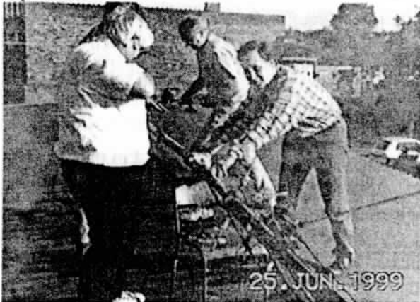
Ken, Ivor and Matthew on the roof at Filton, working on the old 'ZZ antenna stack
